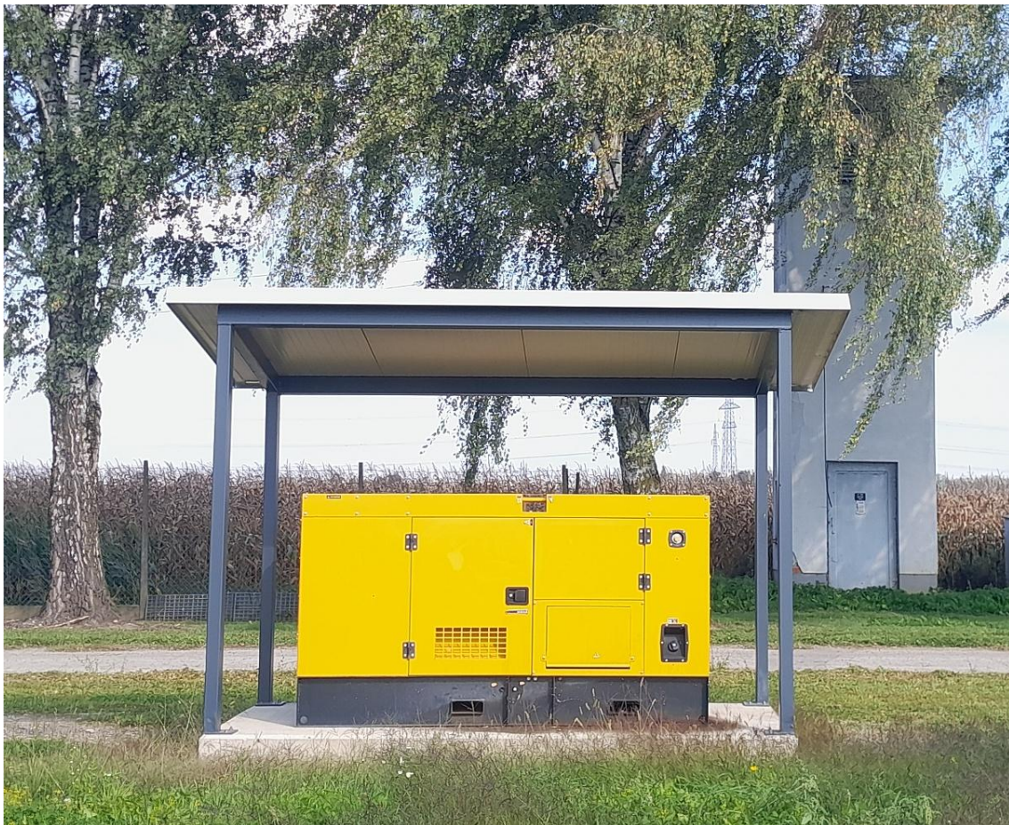
Diesel generator in transformatorska postaja
